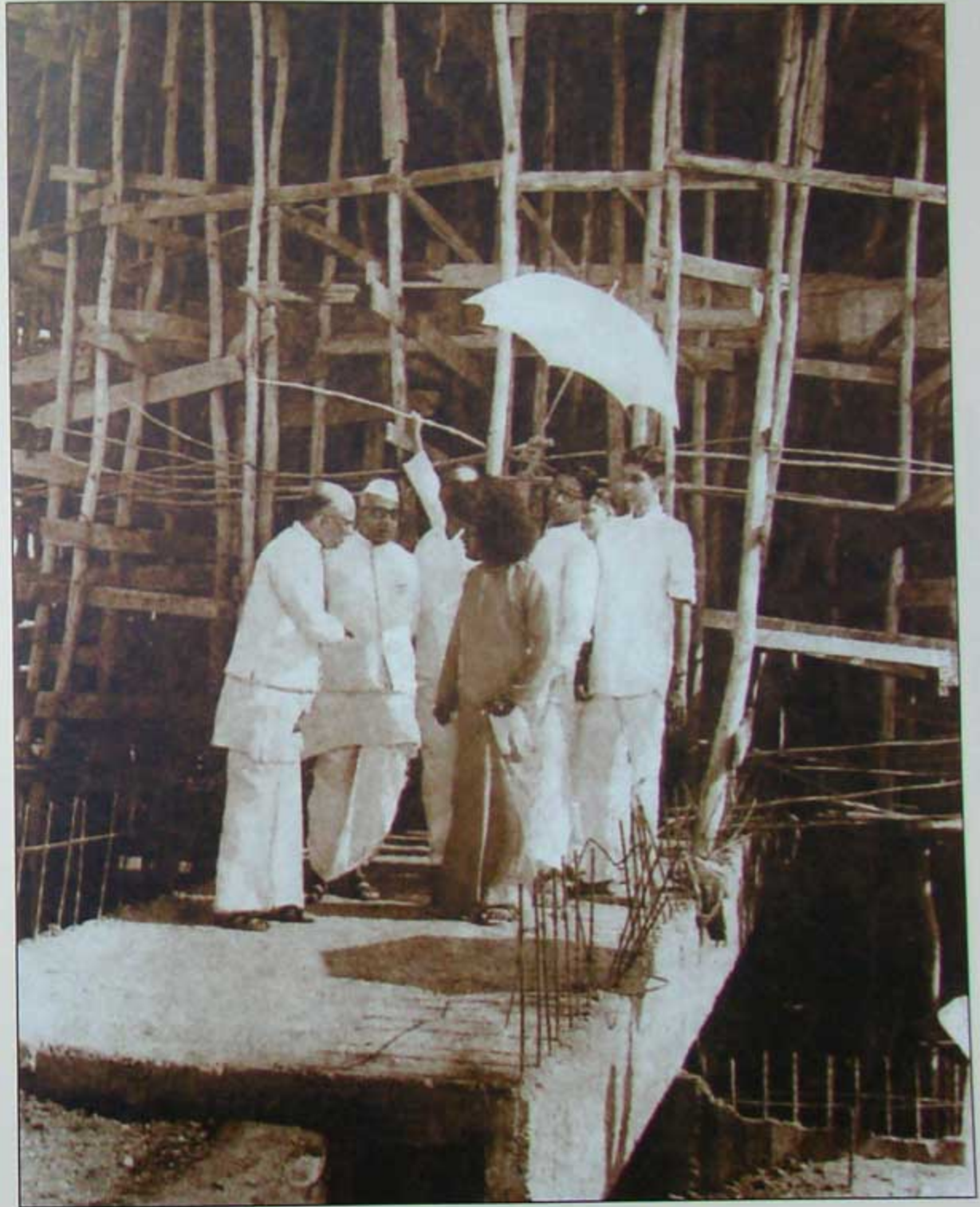
Bhagawan inspecting progress of construction of Sathya Deep
