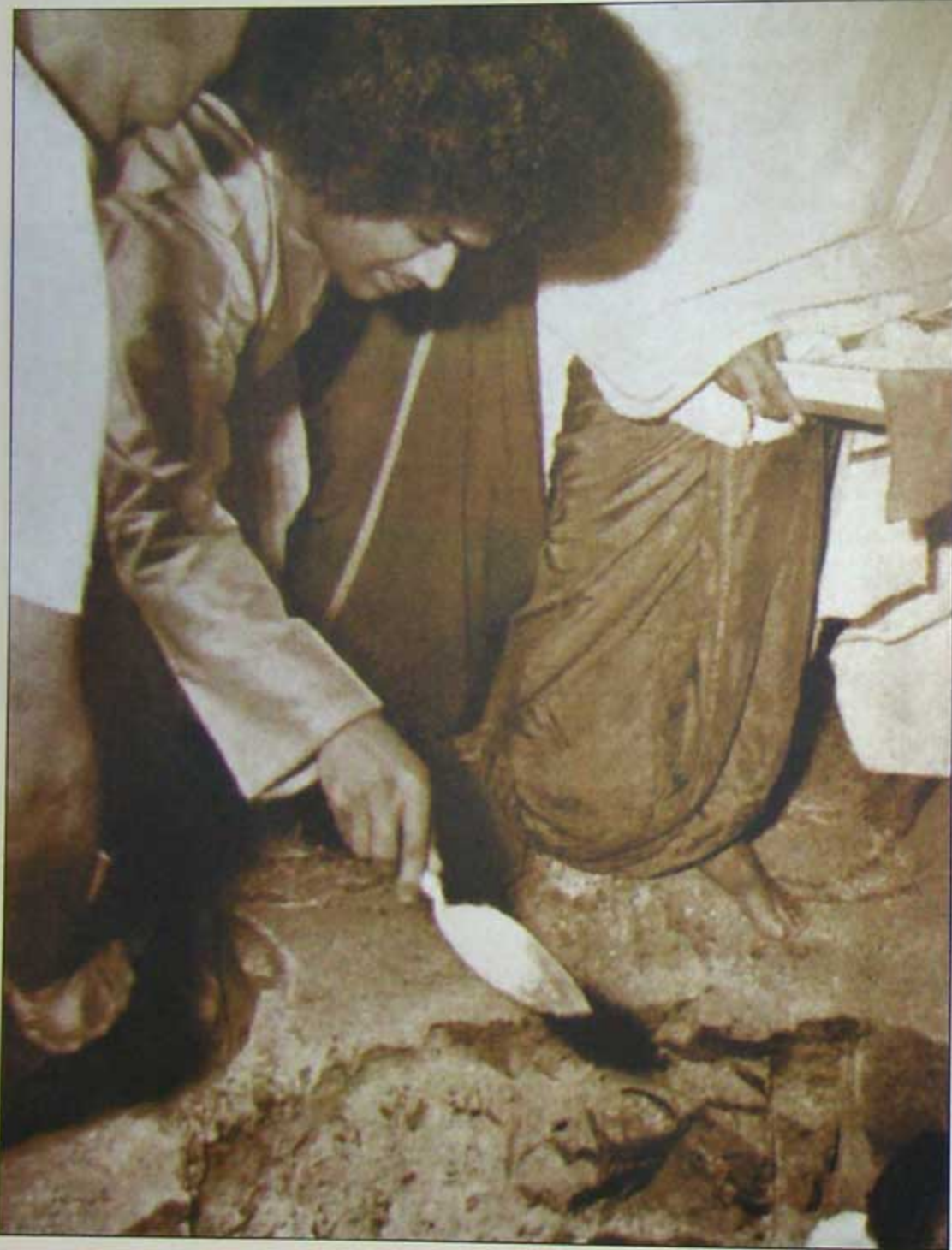
A rare photograph of Bhagawan laying the Foundation Stone of Dharmakshetra on 3 November 1967.
