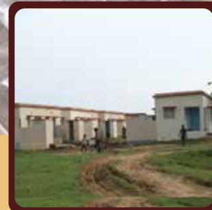
Orissa Flood Rehabilitation Housing Project Second Phase (Rs. 6 Crores)
